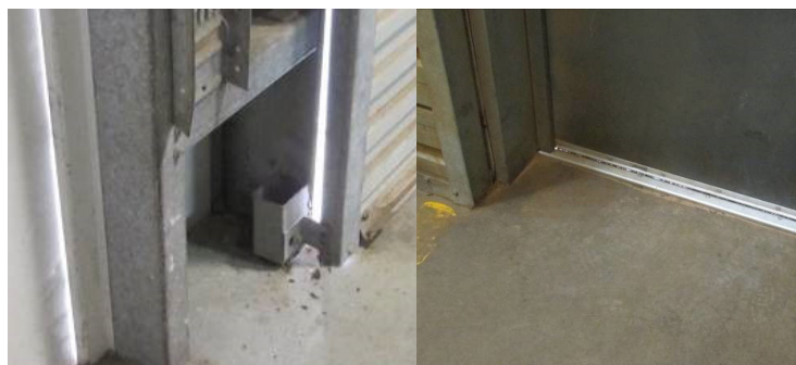
Figure 8: Small holes (>6mm) allow entry into facilities. This is especially important around roller doors where it is difficult to reduce gaps. (a) Small gap alongside roller door allowing entry. (b) Well fitting metal door strips improve management of entry of mice.
